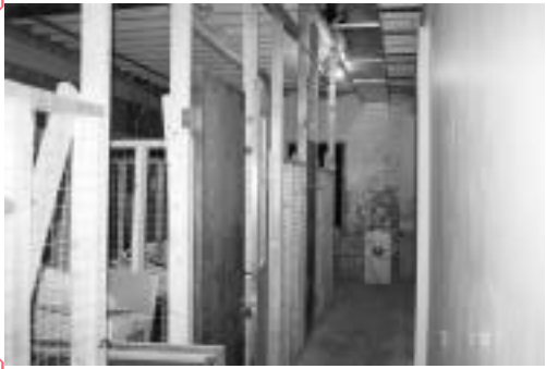
Unfinished storage space prior to remodeling (no lighting, heat, A/C, etc.)
