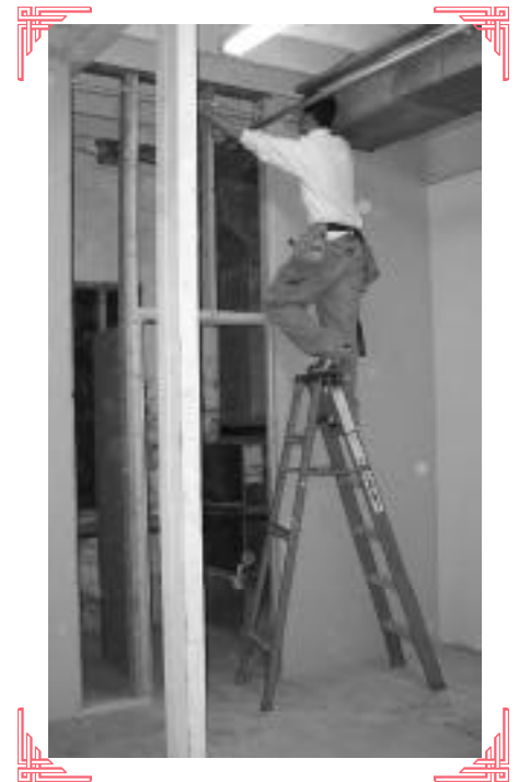
Annex space under construction
