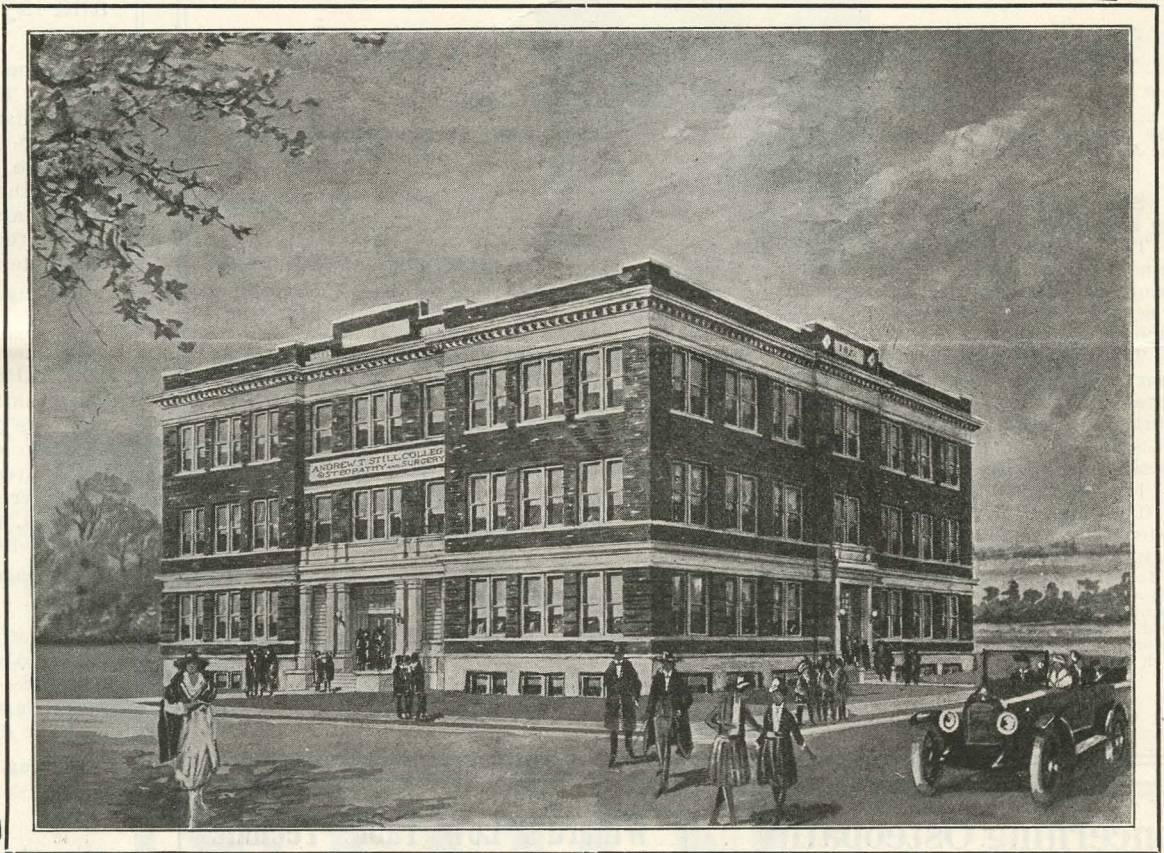
From Architects drawings—Now under course of construction.
