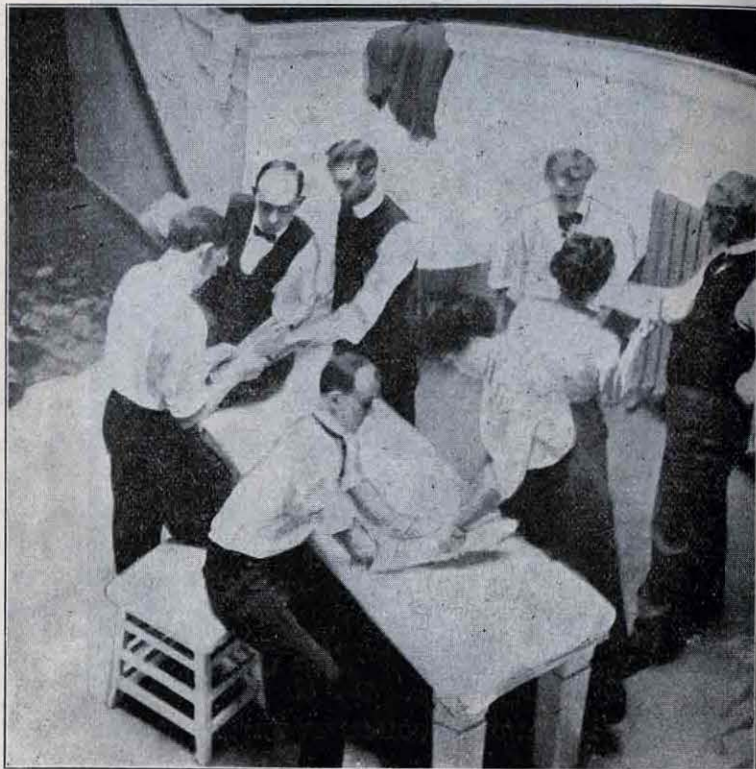
SECTION IN PLASTER BANDAGING WORK IN A. S. O. HOSPITAL
