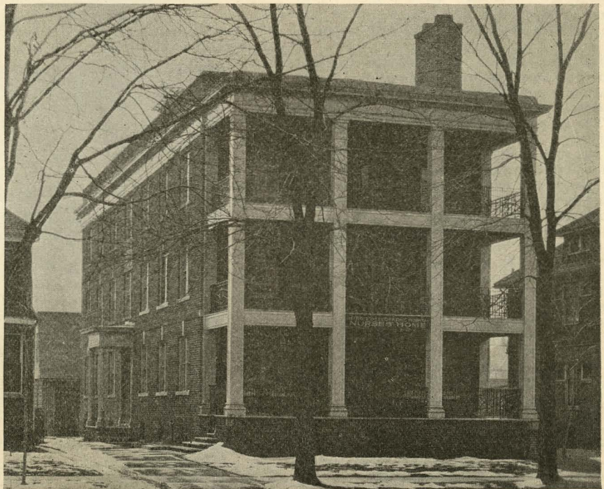
New Osteopathic Nurses' Home at Detroit erected by Mr. Philip H. Gray at a cost of $125,000
